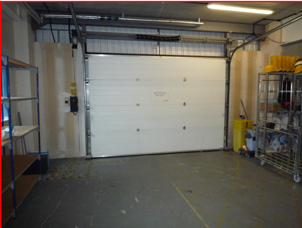
Interior of store area showing the loading door
