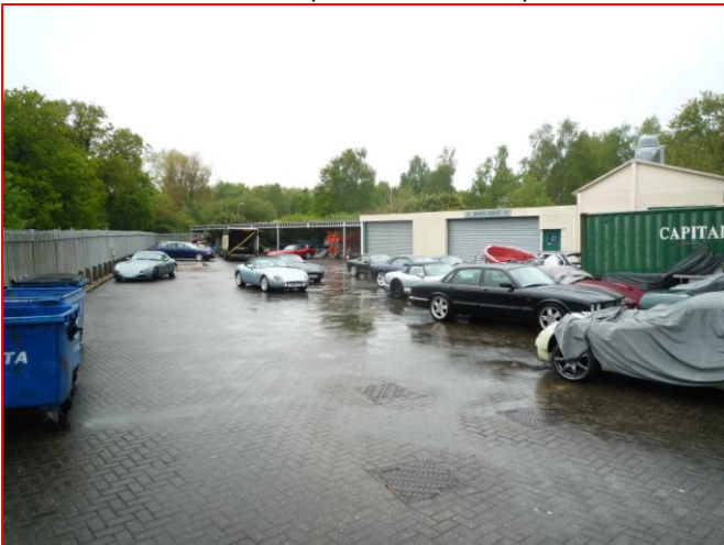
Secure Yard, Covered Storage and Stand Alone Industrial Workshop
