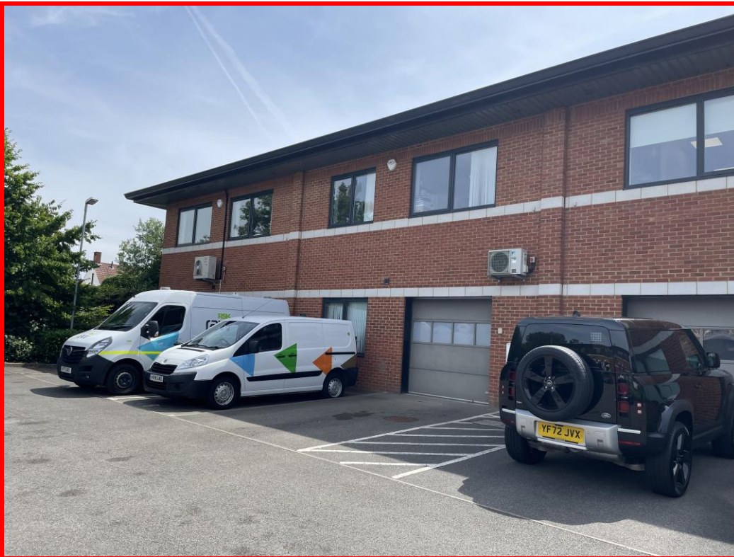
Rear Elevation (middle terrace) showing the loading door
