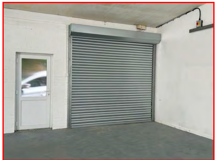
Roller door and main entrance door
