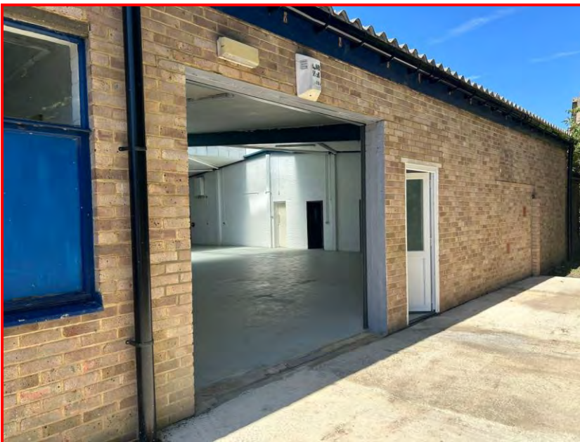
Loading Door Open & Pedestrian Door
