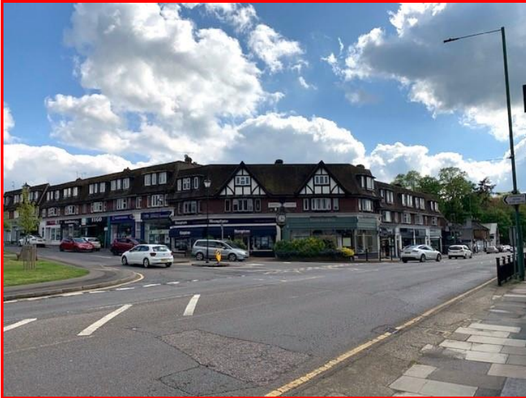
Chobham/London Road junction
