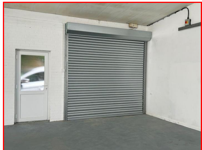
Roller door and main entrance door
